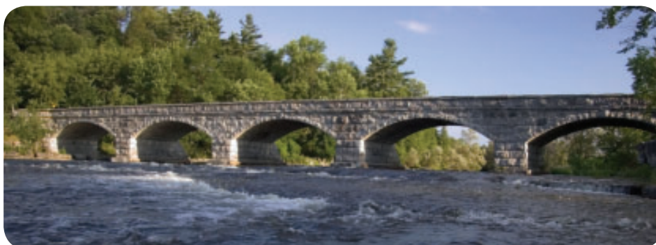
Figure 6 The arch transfers compression force downward from each stone to the next.
